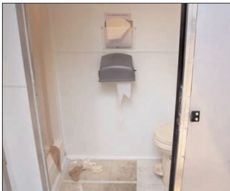
Portable restrooms and showers lacked access
